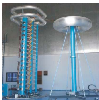
High Voltage laboratory
